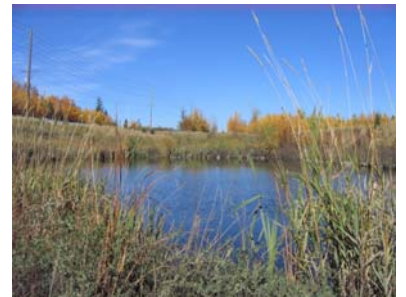
Stormwater detention pond, Westgate Shopping Centre, Prince George, BC
