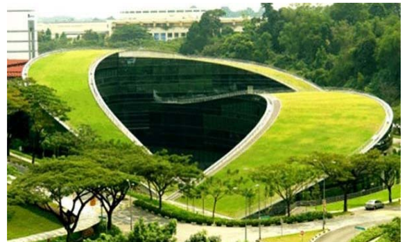
Extensive green roof Nanyang Technological University, Singapore
